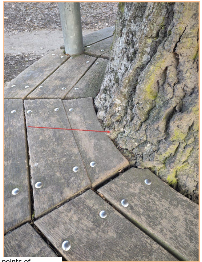
Images showing points of impingement of structure on tree
