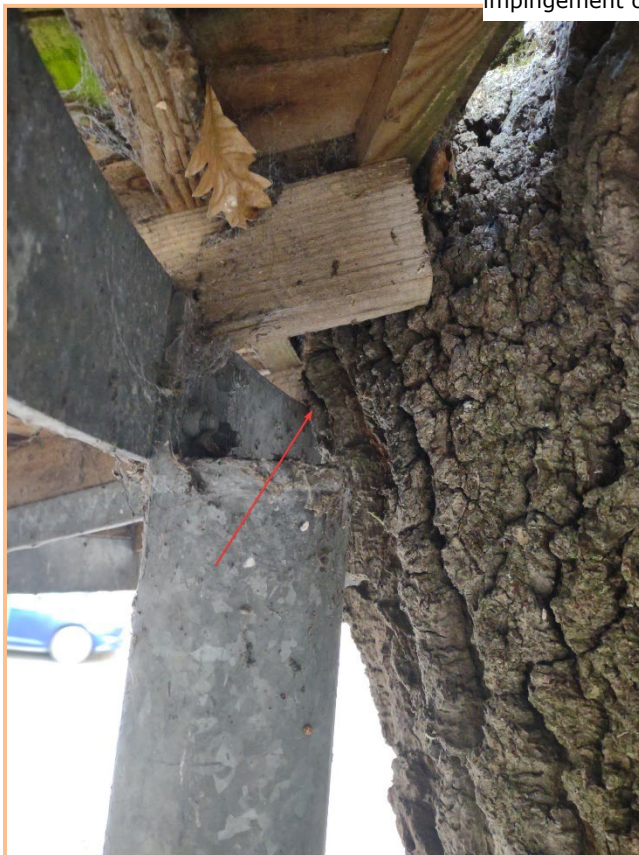
Images showing points of impingement of structure on tree
