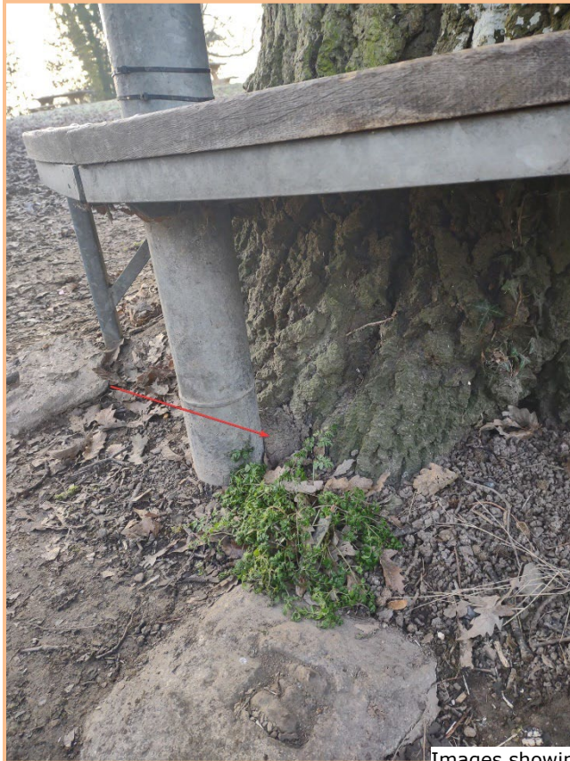
Images showing points of impingement of structure on tree
